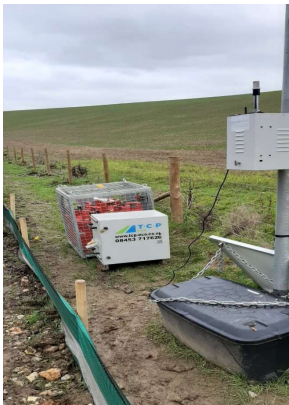
Environmental Monitoring– HS2
